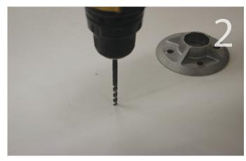
Drill pilot holes for the fasteners based on American Wood Council recommendations. Make sure to drill perpendicular to the roof. Backfill the pilot holes with a sealant compatible with roofing materials.
