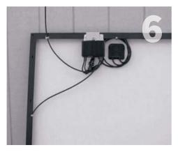
Neatly coil the wires and clip to module frame.
