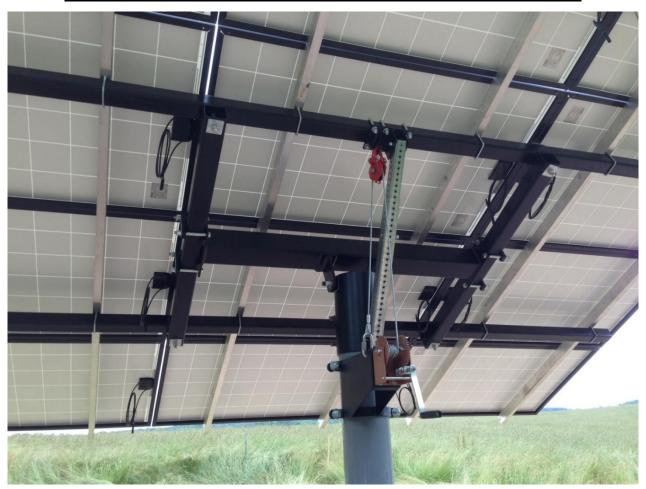
PIVOT CAP: 9 1/4" O.D. 15" TALL PIPE SOCKET
