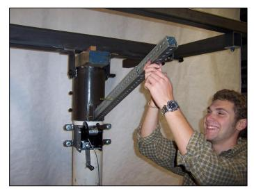
Install the 2 ¼" x 2 ¼" end of telestrut between the lugs on the bottom of the pivot cap. Tighten the nyloc nut all the way.
