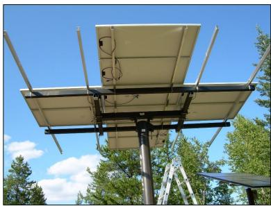
Repeat rail attachment procedure on left and right until all remaining panels are installed. When all panels and spaces are square and even to one another, tighten stainless steel panel bolts and all u-bolt nuts.
