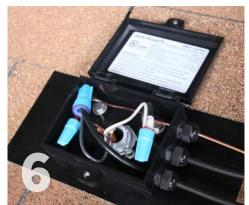
Push Wires Into Box: Push wires down into the box and away from the lid. Lid should close freely without wire interference. Failure to do so will prevent proper rainproofing of the enclosure, voiding the warranty and possibly leading to a short. Secure the lid per step 12 in section IV.
