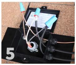
Connect Wires: Install Approved wire connectors. Refer to Section VI for allowable wiring combinations.
