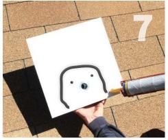
Optional Caulk: Apply an upside down U-shaped bead of sealant to the underside of the flashing before insertion. Do not use excessive sealant.
