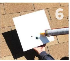
Caulk: Fill the fastener holes with appropriate sealant.
