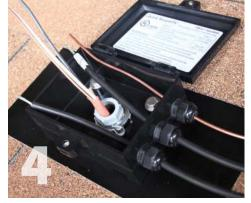
Install Output Wires: Transition wires may have pulled when the transition fittings were installed. If not, do so now, and label all wires appropriately. Strip sheathing from the end of all wires per instructions found in Section VI. Ensure each wire has a minimum of 6" of lead inside the box.
