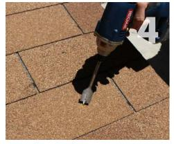
Drill Conduit Hole: Remove QBox flashing and drill 1" hole at location marked in Step 3. Use either a spade bit or hole saw. Avoid all electrical components on underside of deck in the attic.
