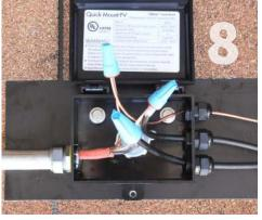
Connect Wires: Pull min 6" of transition wiring into the QBox, label all wires, and strip sheathing from the end of all wires per the instructions of the manufacturer of the connectors being used. Follow step 6 to complete the installation.
