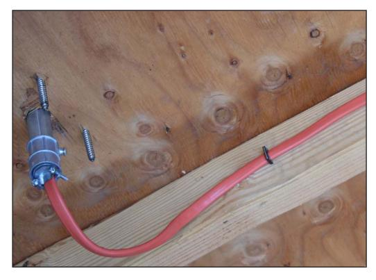
**Building wiring strapping:** Per the NEC, wire or conduit must be secured within 12" of leaving the QBox conduit nipple. (EMT can be 3')
