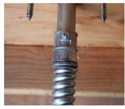
**3/4" Flexible Metal Conduit:** -3/4" EMT QBox Conduit Nipple -3/4" EMT to 3/4" NPT threaded coupler (Arlington #2411) -3/4" Knockout Flex fitting (Halex #20442) -3/4" Flexible Metal Conduit
