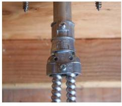
**Double MC:** -3/4" EMT QBox Conduit Nipple -3/4" EMT to 3/4" NPT threaded coupler (Arlington #2411) -3/4" to 1/2" Reducing Bushing (Halex #91321) -1/2" Knockout duplex fitting (Halex #21580) -Double MC
