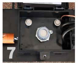
Holes for Conduit: Use the drill starter along the perimeter of the box to guide your hole saw specified by the conduit hub manufacturer. Clean off all burs. Attach the conduit to the box. Ensure that conduit cap and blank are installed.
