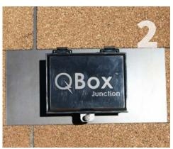
Slide the QBox flashing up underneath the second course of shingles, so that the bottom edge of the flashing does not overhang the front edge of the shingle and the top edge extends up into the third course of shingles.
