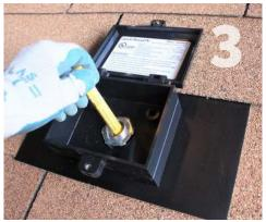
Mark Conduit Location: If not using attic conduit exit, complete only step 6-8 and 11-12. Otherwise, remove the conduit cap and blank and set aside. mark the location to drill the conduit passthrough with a lumber crayon or other marking device.
