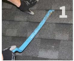
Remove Nails: Use roofing bar to break seals between 1st and 2nd and 3rd shingle courses. Be sure to remove any obstructing nails to allow correct placement of the QBox.
