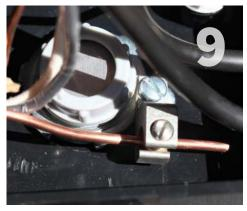
Ground: Since the QBox is non conductive, it does not need to be grounded. However, for NM style connections or if required by an AHJ, a ground wire termination can be accomplished by installing a grounding lug on the conduit lock ring using the bolt provided.
