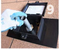
Install Conduit: Install the supplied conduit nipple through the QBox and the roof with the flared end facing up.
