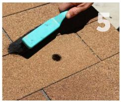
Clean: Clean debris from roof to ensure the flashing is as flat as possible against the roof surface and clean for adhesion.
