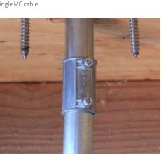
**3/4" EMT:** -3/4" EMT QBox Conduit Nipple -3/4" EMT to 3/4" EMT coupler (HALEX # 26282) -3/4" EMT
