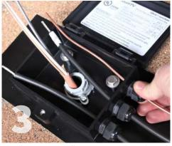
Install PV Wires: Pull PV system wiring through the cord grips and tighten the cord grips to seal around the wires making a watertight connection. Ensure each wire has a minimum of 6" of lead inside the box per NEC requirements.
