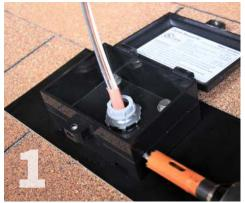
Holes for Cord Grips: Use the drill starter along the perimeter of the box to guide your hole saw. Hole size is specified by the cord grip or conduit hub manufacturer. Clean off all burs.
