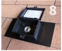
Reinstall Flashing: Reinstall the QBox assembly such that the conduit fitting in the center of the box aligns with the hole you created in step 4.
