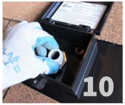
Finish Conduit Attach: Hand tighten threaded conduit cap to secure conduit nipple in place. This will hold the QBox flashing in place when securing it to the roof.
