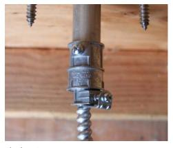
Single MC: -3/4" EMT QBox Conduit Nipple -3/4" EMT to 3/4" NPT threaded coupler (Arlington #2411) -3/4" to 1/2" Reducing Bushing (Halex #91321) -1/2" Knockout MC fitting (Halex #20670) -Single MC cable
