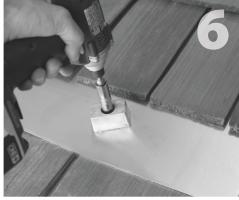
Slide mount into position. Prepare hanger bolt with 1 hex nut (item 5) and 1 sealing washer (item 9). Insert bolt into QBlock hole and drive into rafter, tightening until the QBlock no longer swivels easily.
