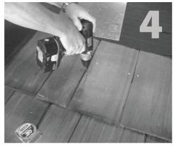
Set mount aside. Using drill with 7/32" bit, drill pilot hole into roof and center of rafter, taking care to drill square to the roof. Do not use mount as a drill quide.
