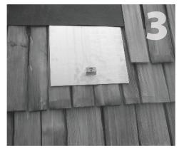
Level out any high spots beneath the flashing area with a grinder or sander. Slide mount into desired position on shakes, under felt paper, and mark center for drilling with a pen or pencil.\*
