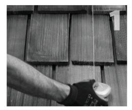
Locate, choose, and mark centers of rafters to be mounted. Select the courses of roofing where Quick Mounts will be placed.
