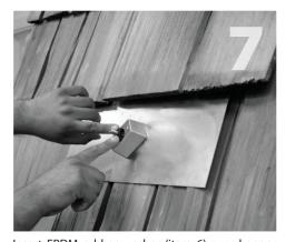
Insert EPDM rubber washer (item 6) over hanger bolt into QBlock.
