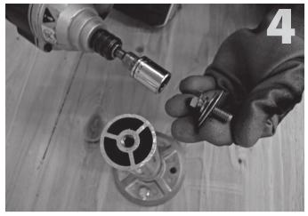
Attach the hardware (items 5-8) to the top of the post. (Be sure to seal off the post from weather exposure with the sealing washer (item 5), in the interim before racks are installed.) You are now ready to flash the mount, roof around it, and attach racking. Aluminum flashings for built-up roofs are available from Quick Mount PV in 4" and 8" cones (sold separately). For membrane roofs, be sure to use manufacturer-specified flashing and utilize the services of a certified roofer.
