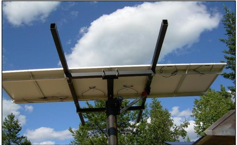
Center rails on longitudinals by equally measuring side to side to longitudinal ends. Then place the rest of the panels on the rails. NOTE: Leave the bolts on the PV panels screwed together but loose for now.
