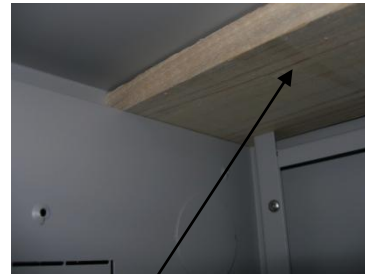
3/4" Piece of wood added as support
