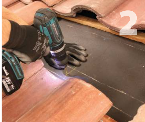
2 Rest the base plate over center of rafter and mark center of holes. Drill two 7/32" pilot holes and fill with sealant compatible with roofing materials.
