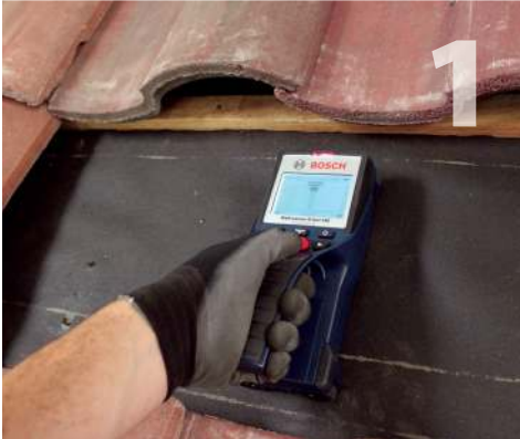
1 Remove the tile at selected location of the mount. Locate and mark the center of the rafter.
