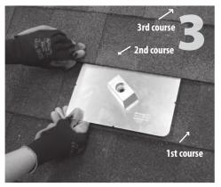
Insert flashing between 1st and 2nd course. Slide up so top edge of flashing is at least 3/4" higher than the butt-edge of the 3rd course and lower flashing edge is above the butt-edge of 1st course. Mark center for drilling.
