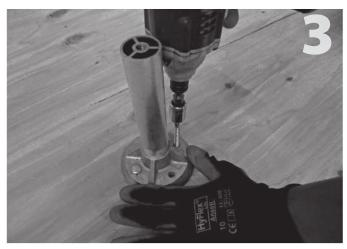
Prior to attaching the base to the roof, place the grade-8 hex bolt (item 1) in the bottom of the base (item 2) and screw the post (item 4) in. This is easier than adding the post after securing the base to the roof. Attach the base/ post assembly to the roof with two lag bolts (item 3).
