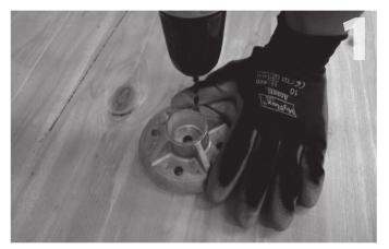
Locate the desired mount placement over a rafter (or custom wood blocking). Using the base as a template, mark the two penetration points with either a pen or light drilling. Use two opposing holes on the base plate, parallel to the structural member.
