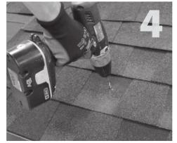
Using drill with 7/32" bit, drill pilot hole into roof and rafter, taking care to drill square to the roof. Do not use mount as a drill guide. Drill should be 'long style bit' aka 'aircraft extension bit' to drill a 3" deep hole into rafter.
