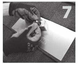
Insert EPDM rubber washer over hanger bolt into block.
