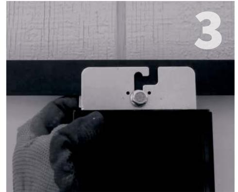
Slide this assembly onto the module frame with the bracket behind the module frame, the module level electronic mounting bracket in front of the module frame.
