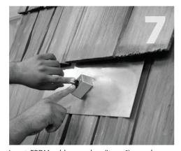
Insert EPDM rubber washer (item 6) over hanger bolt into QBlock.
