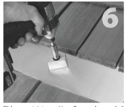
Slide mount into position. Prepare hanger bolt with 1 hex nut (item 5) and 1 sealing washer (item 9). Insert bolt into QBlock hole and drive into rafter, tightening until the QBlock no longer swivels easily.
