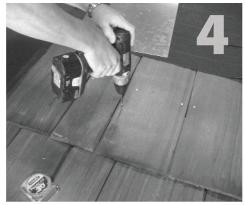
Set mount aside. Using drill with 7/32" bit, drill pilot hole into roof and center of rafter, taking care to drill square to the roof. Do not use mount as a drill quide.
