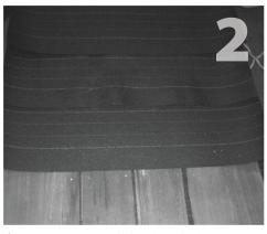
If necessary, remove shakes directly above mount with the roofing bar to expose felt paper. Flashing should reach at least 1 inch up and under the felt paper for proper waterproofing.
