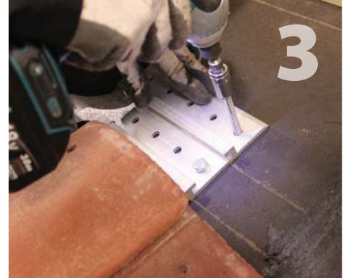
Connect hook to base plate and drive lag screws into rafter through the two holes to a solid, snug fit. DO NOT over tighten lag screws, this may compromise their holding strength.
