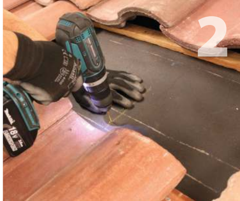
Rest the base plate over center of rafter and mark center of holes. Drill two 7/32" pilot holes and fill with sealant compatible with roofing materials.
