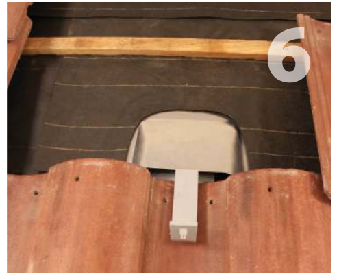
Waterproof at underlayment level according to roofing manufacturer instructions and Tile Roofing Institute Guidelines.
