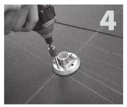
Fill pilot holes with sealant compatible with roofing material. Seat grade 8 cap screw through bottom of QBase. Place QBase over drilled holes and secure lags in place, to a solid, snug fit.
