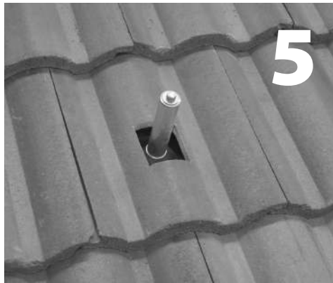
With a diamond blade on a grinder or skill-saw, cut tile to allow post to pass through. Place cut tile back in position. Insert post and tighten into place.
