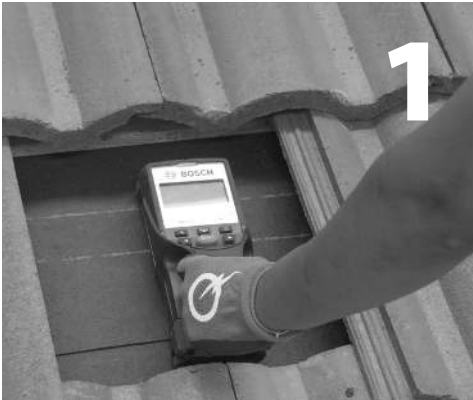
Remove tile. Locate and mark center of rafter.
