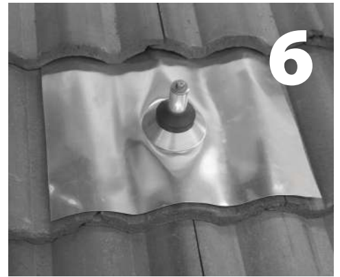
Install the 18"x 18" flashing. Pre-bend the flashing to follow the contour of the tile if curved. Apply sealant where post and flashing meet, and install EPDM counter flashing collar. Seal off the post from weather exposure with the racking hardware in the interim before racks are installed.
