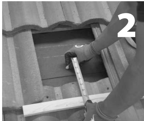
Use a straight edge and measure up 6 5/8" from bottom of tiles to center of the mount over the center of rafter.
