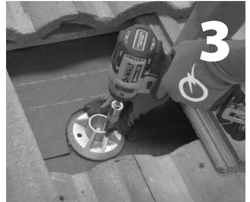
Align QBase over rafter center and drill two 7/32" pilot holes. Fill pilot holes with sealant compatible with roofing material. Place grade-8 cap screw under QBase in hex slot, threads pointing up. Lag QBase into rafter through pilot holes.
